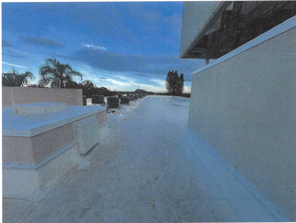
Figure 2: Roof Deck, view to S.
