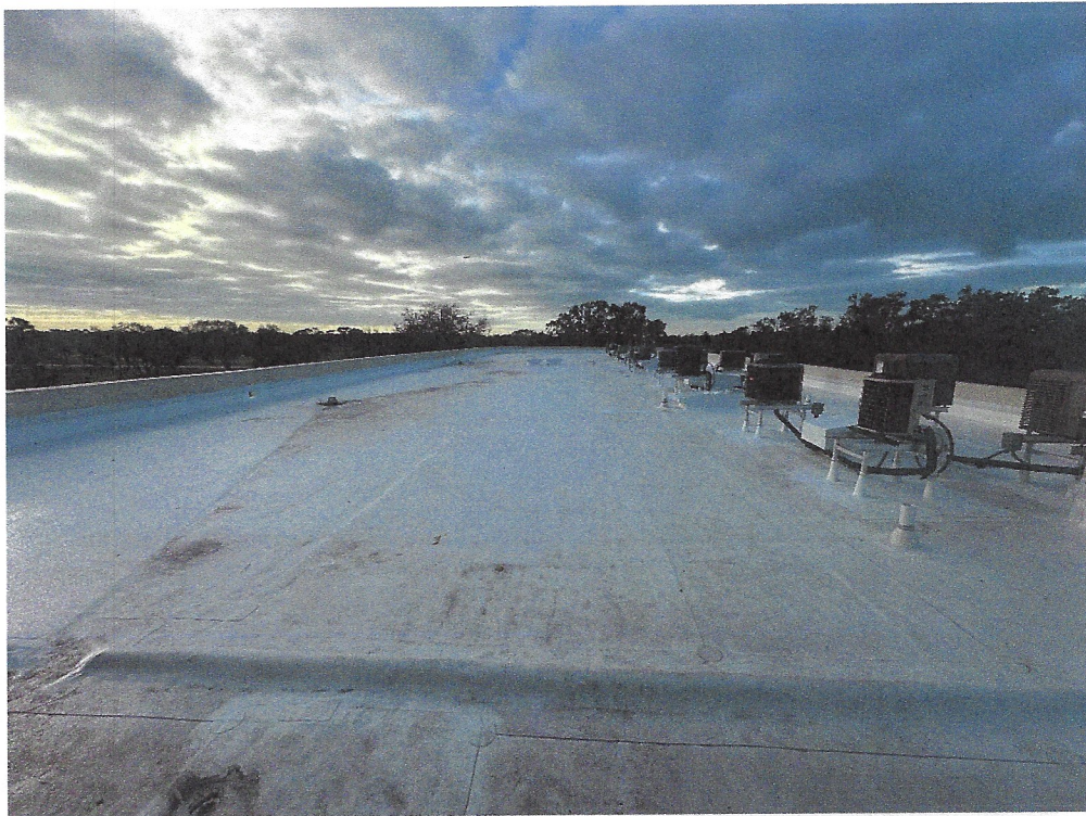
Figure 1: Roof Deck, view to N.
